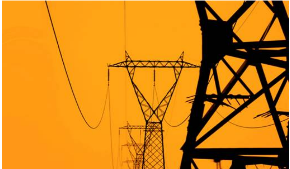
The PUD is installing 168 miles of fiber optic cable and upgrading 62 substations as part of a major "smart grid" system upgrade.
